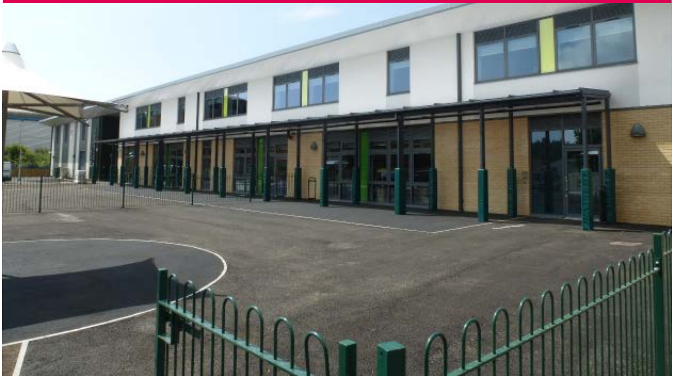
Recent new build primary school in Cardiff - Ysgol Glan Morfa
